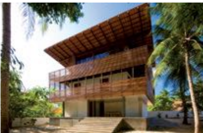
Category F - Rehabilitation & reconstruction 3rd Prize: Vasco Matias Correia and Patricia Sousa (Portugal). Tropical House
